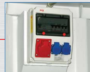
distribution box with integrated sockets
